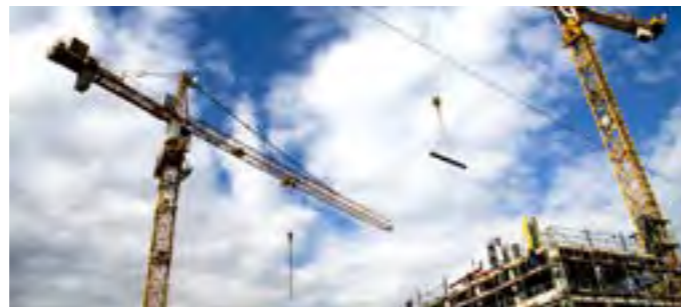
ŞANTİYELER / BUILDING SITE
